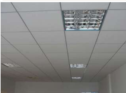
Suspended Ceiling Works
